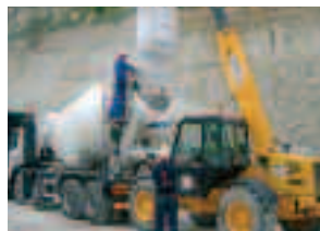
With ready-mix truck
