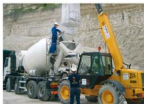
With ready-mix truck
